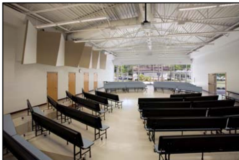
Loften High Classroom & Multipurpose Building / Interior of Multipurpose Room
