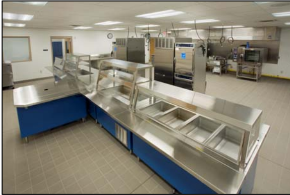
Loften High Classroom & Multipurpose Building / Interior of Kitchen
