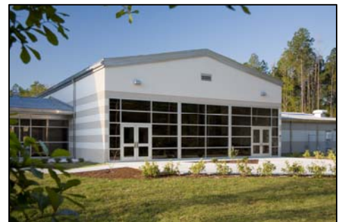
Exterior of rear of Multipurpose Room
