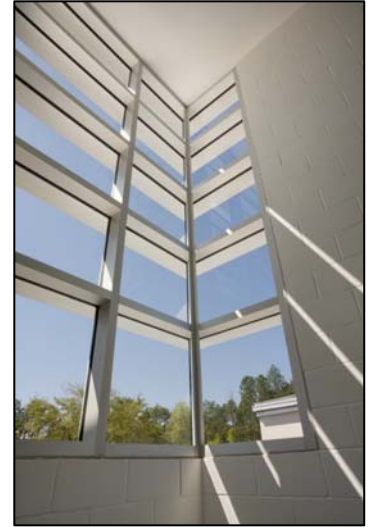
Interior of Stairs
